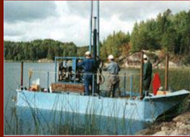
Water Boring from Barge for Bridge Crossing
