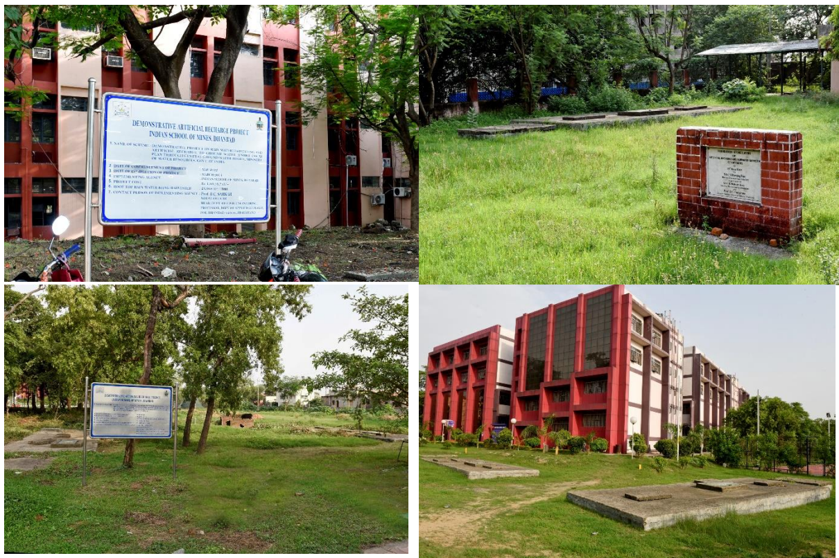
Fig 1: Photographs of Rain water Harvesting pits at IIT(ISM) Dhanbad
