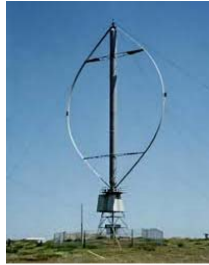
Darrieus straight blade wind turbine
